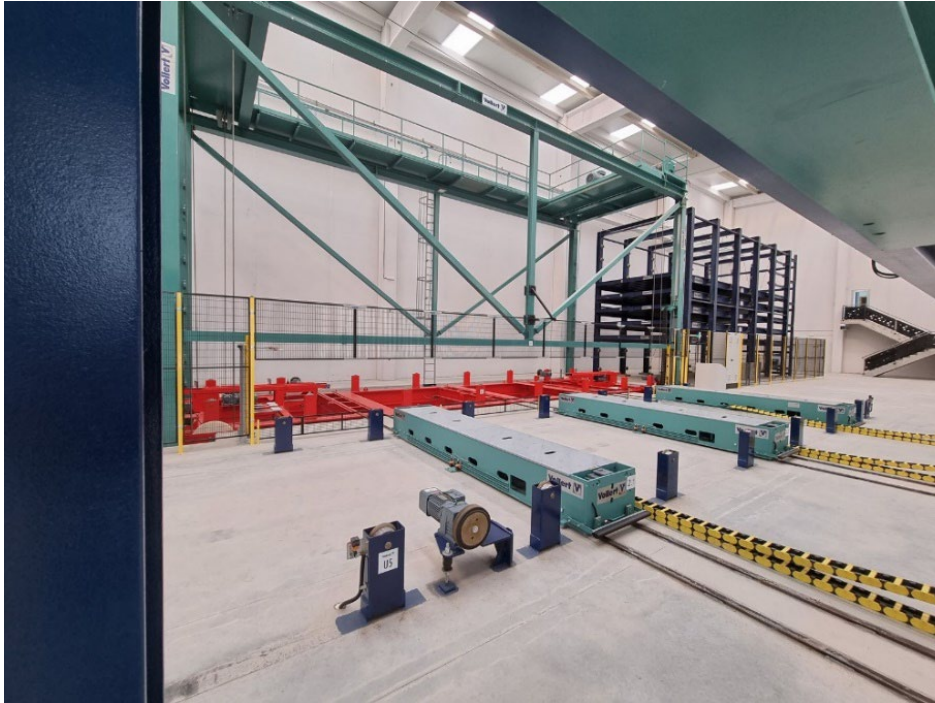
Image 5: A VARIO CURE curing chamber with two rack towers and 10 curing stations each ensures the curing process.
